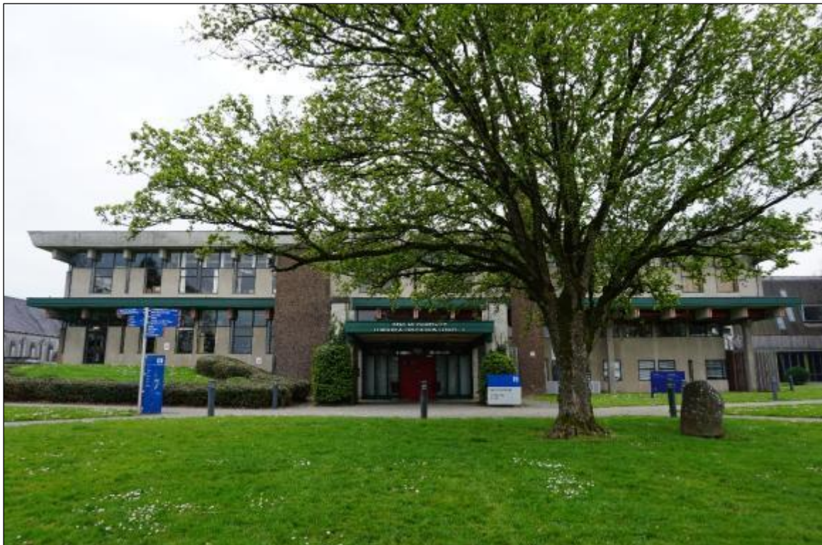
Photograph 13 Library front elevation
