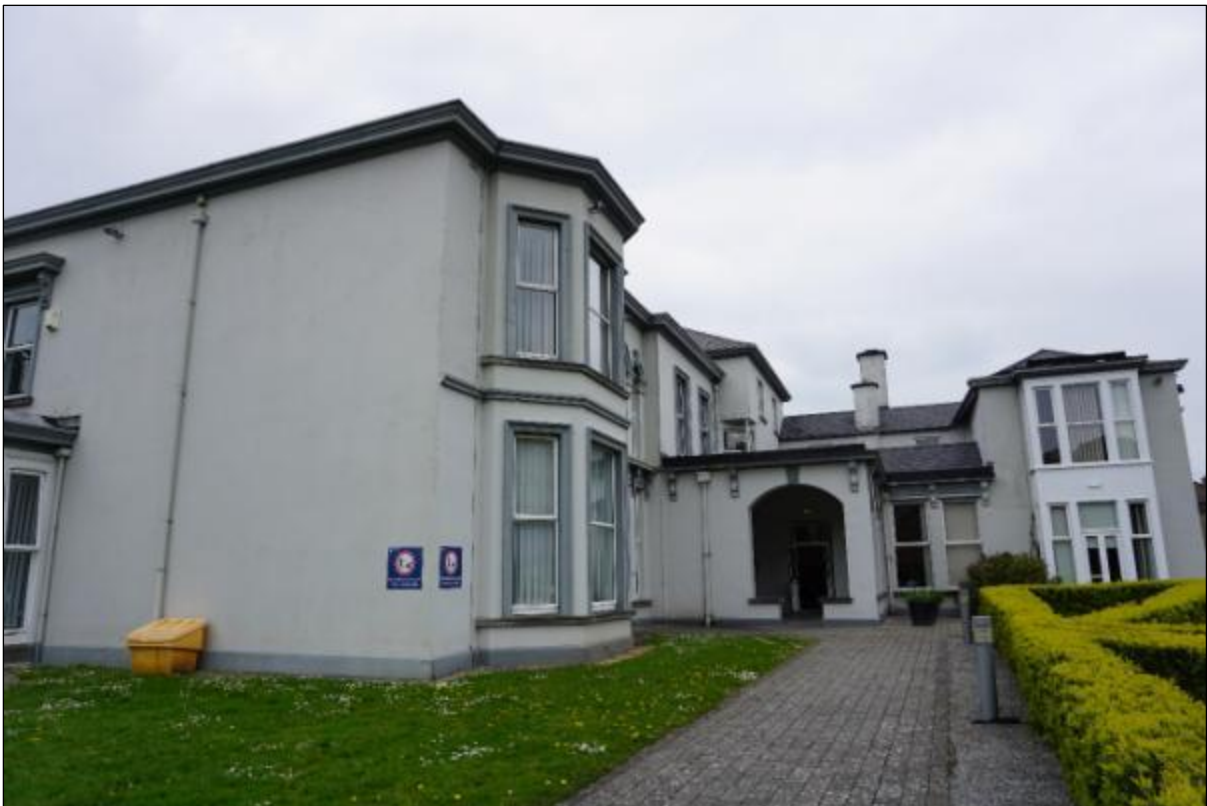
Photograph 86 Rear entrance facing the main buildings on campus.
