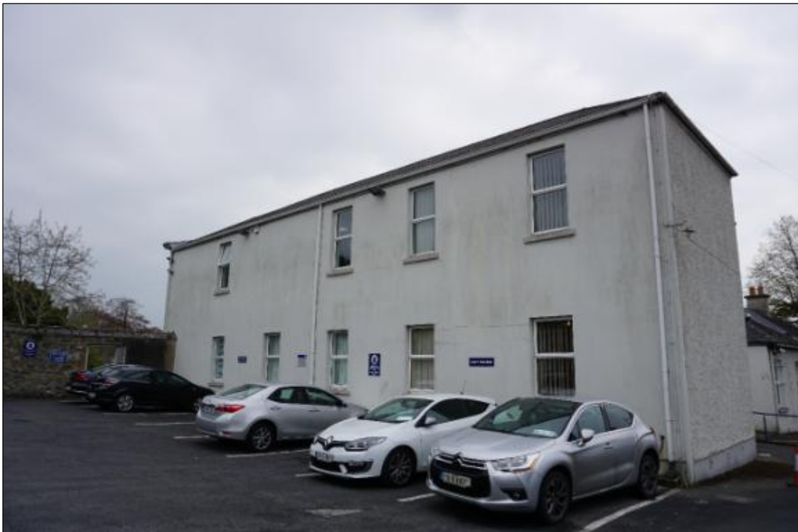
Photograph 21 Rear Elevation of Summerville House
