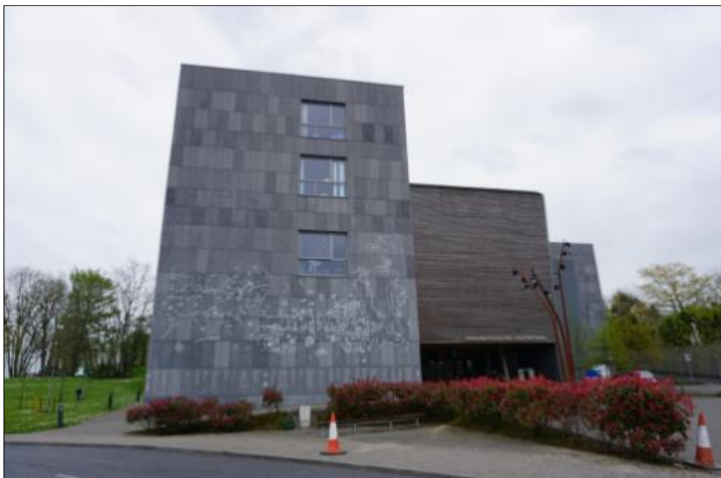
Photograph 17 TARA Building and Lime Tree Theatre Entrance
