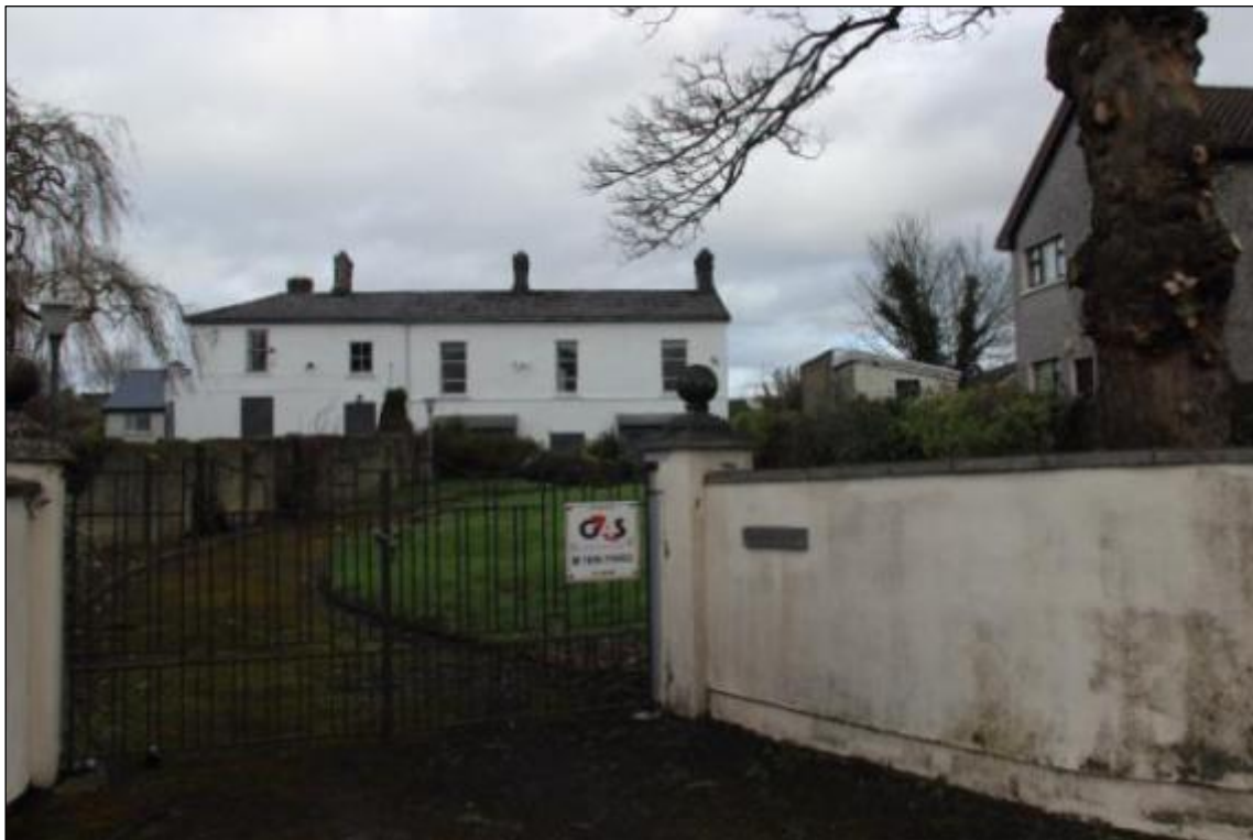
Photograph 26 Richmond and Hillsborough House(s)
