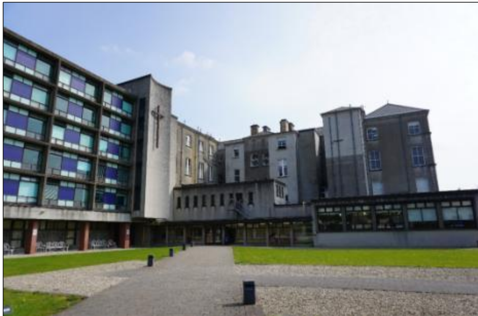
Photograph 4 Rear Elevation of Foundation Building showing additions
