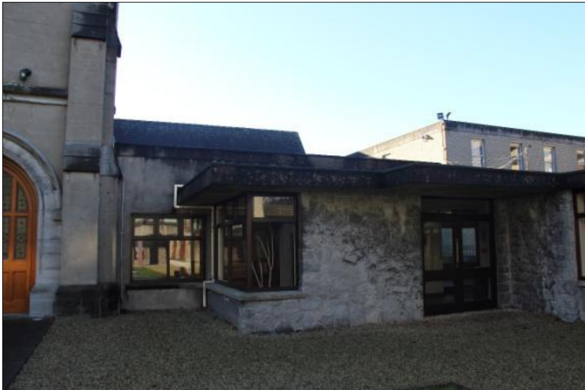
Photograph 10 Single Storey addition next to Chapel
