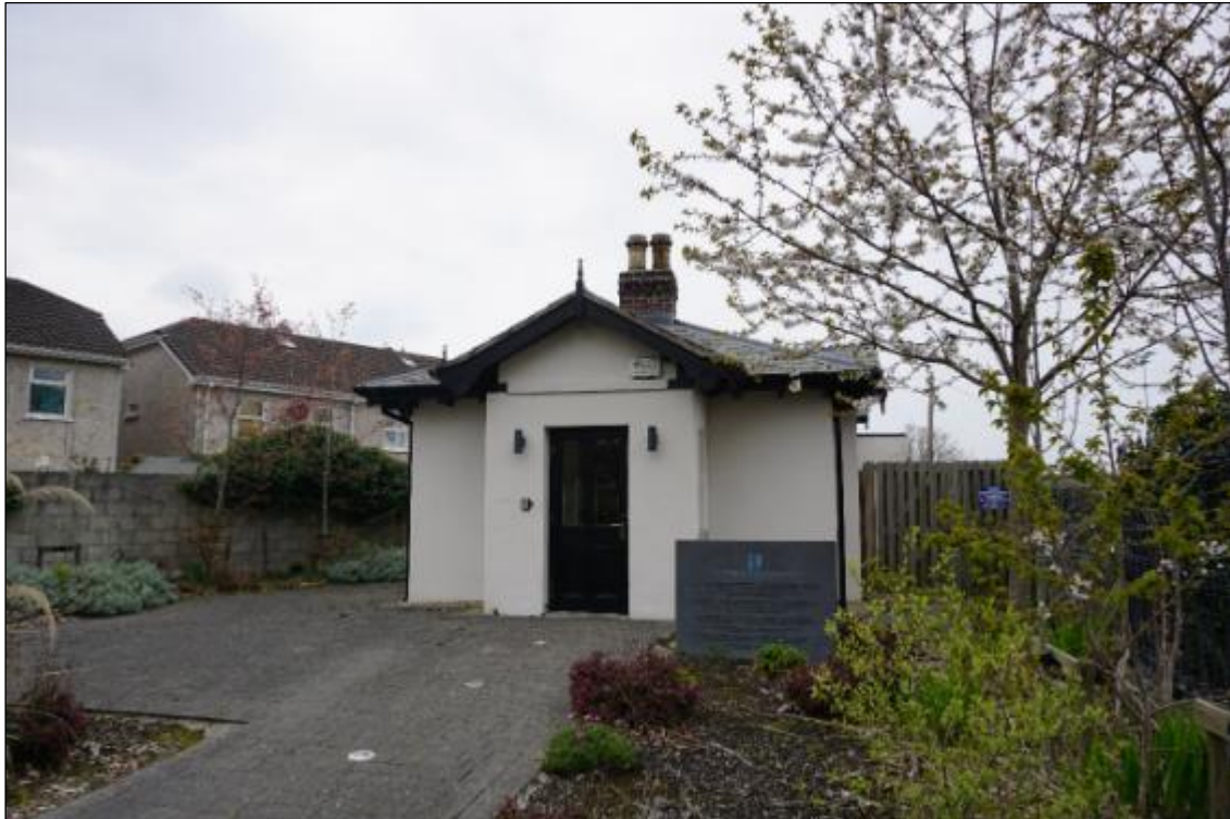
Photograph 97 Summerville Lodge Front Elevation
