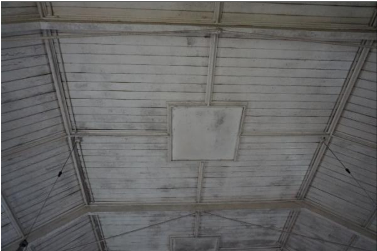
Photograph 118 View of boarded ceiling
