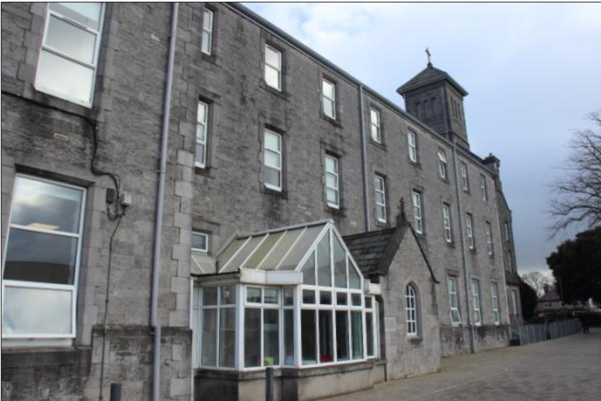
Photograph 102 Side Elevation of Mount St. Vincent
