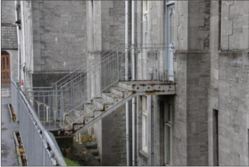
Photograph 105 The Nine Steps
