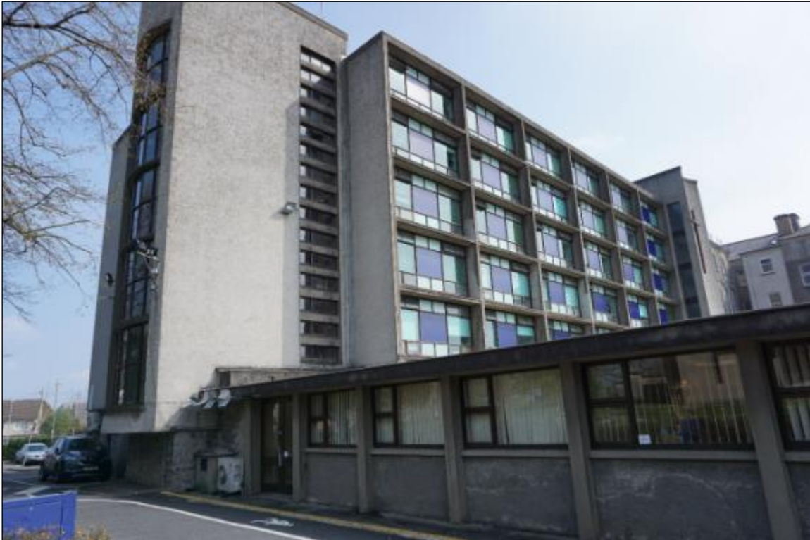
Photograph 11 Single Storey addition next to Residential Block
