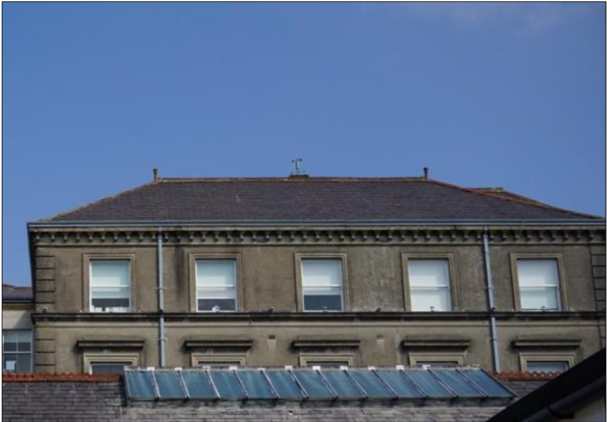
Photograph 67 Mary I foundation Building Side View
