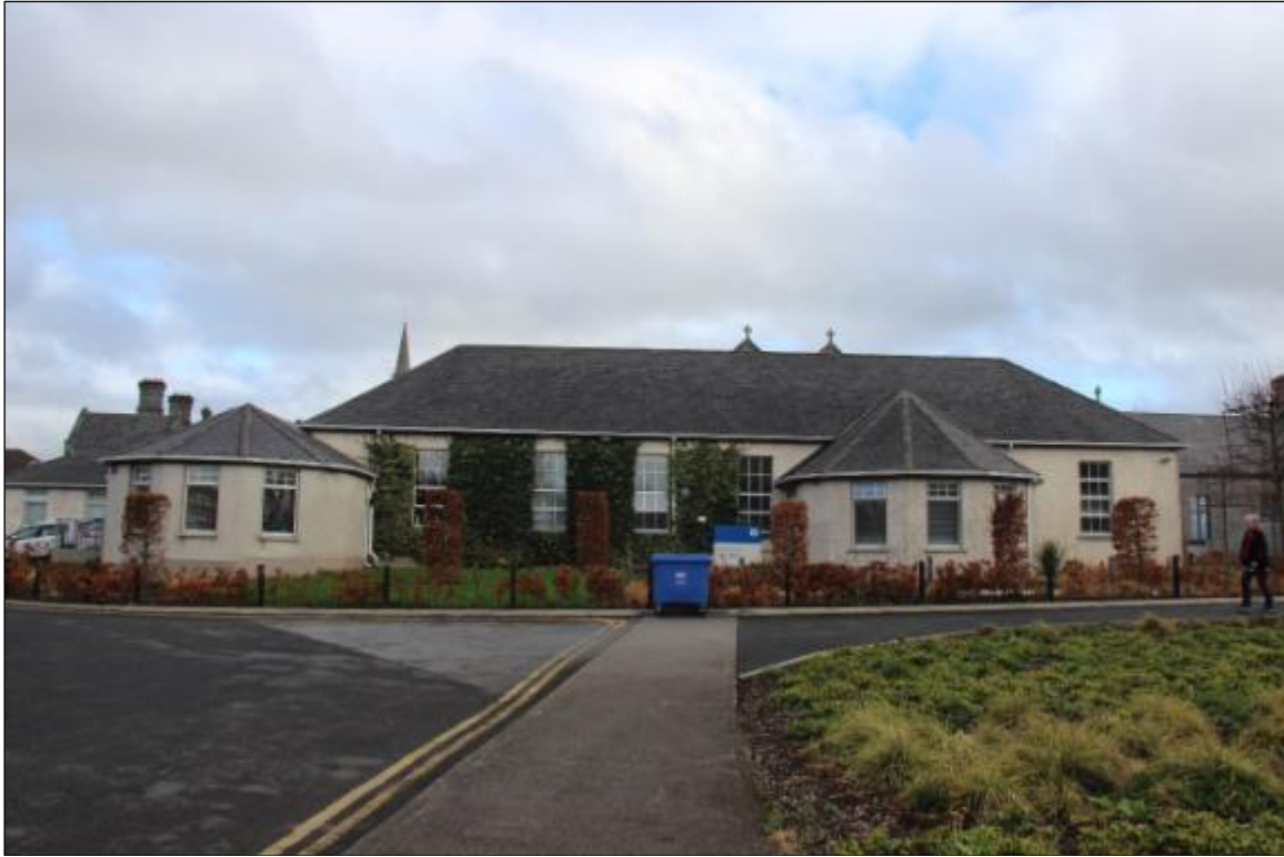
Photograph 27 Gerard House Front Elevation
