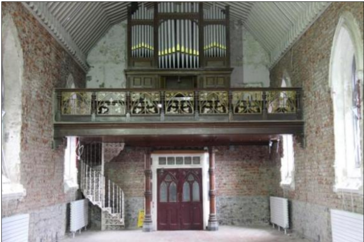
Photograph 111 Interior View of Chapel
