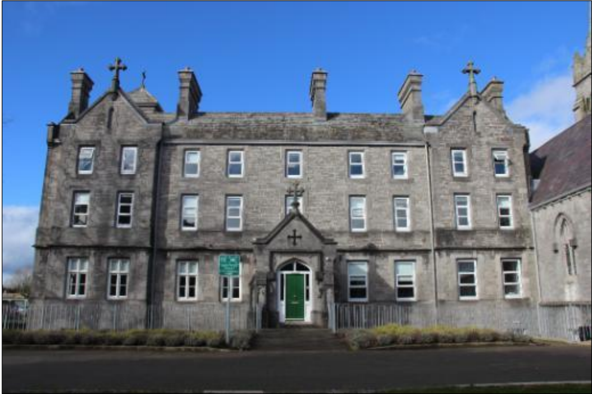
Photograph 29 Mount St. Vincent Front Elevation
