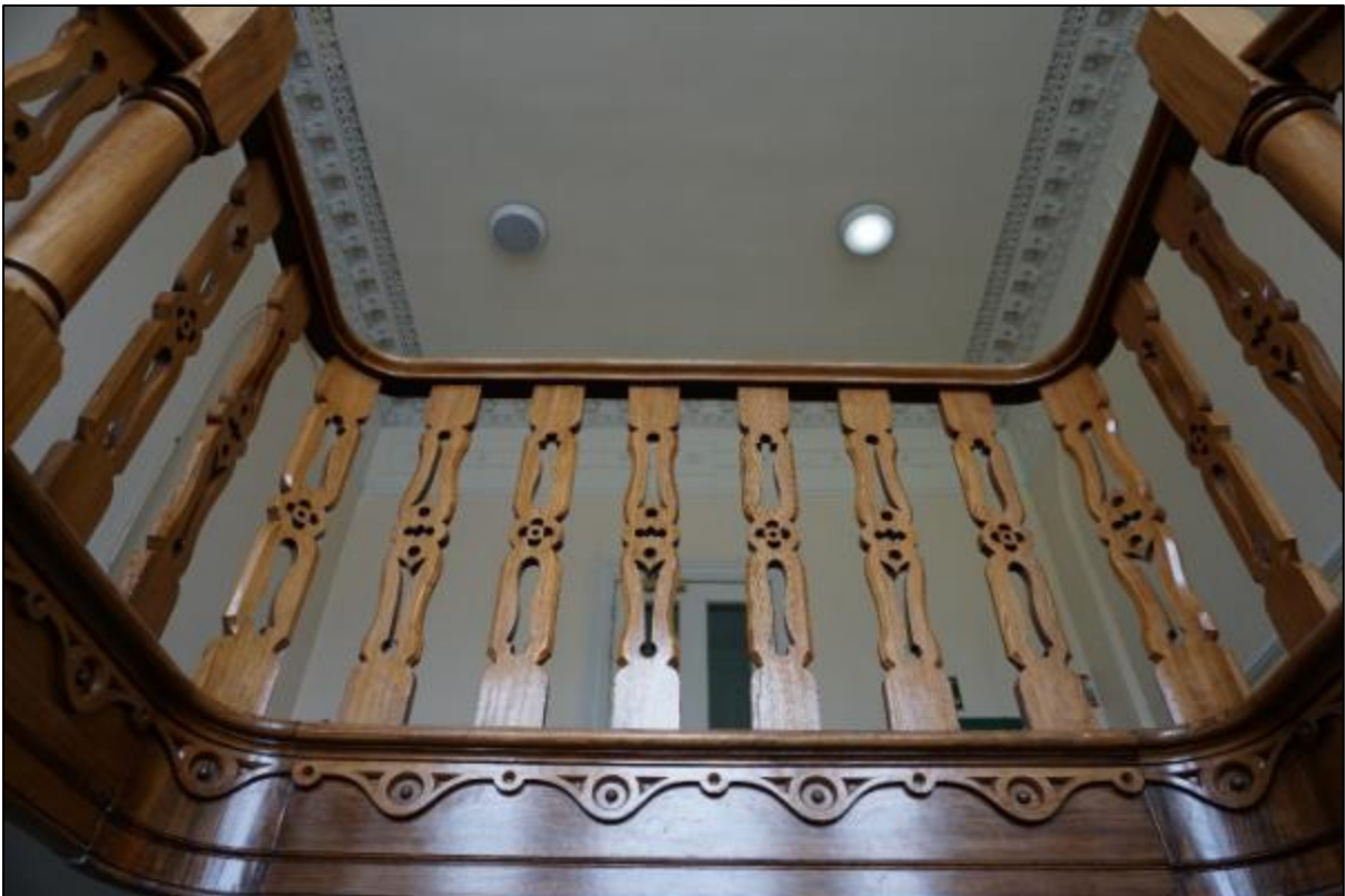
Photograph 94 Railing detailing on main stairs
