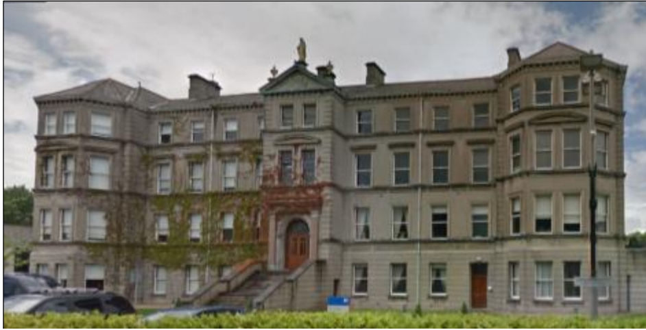
Photograph 3 Foundation Building Front Elevation
