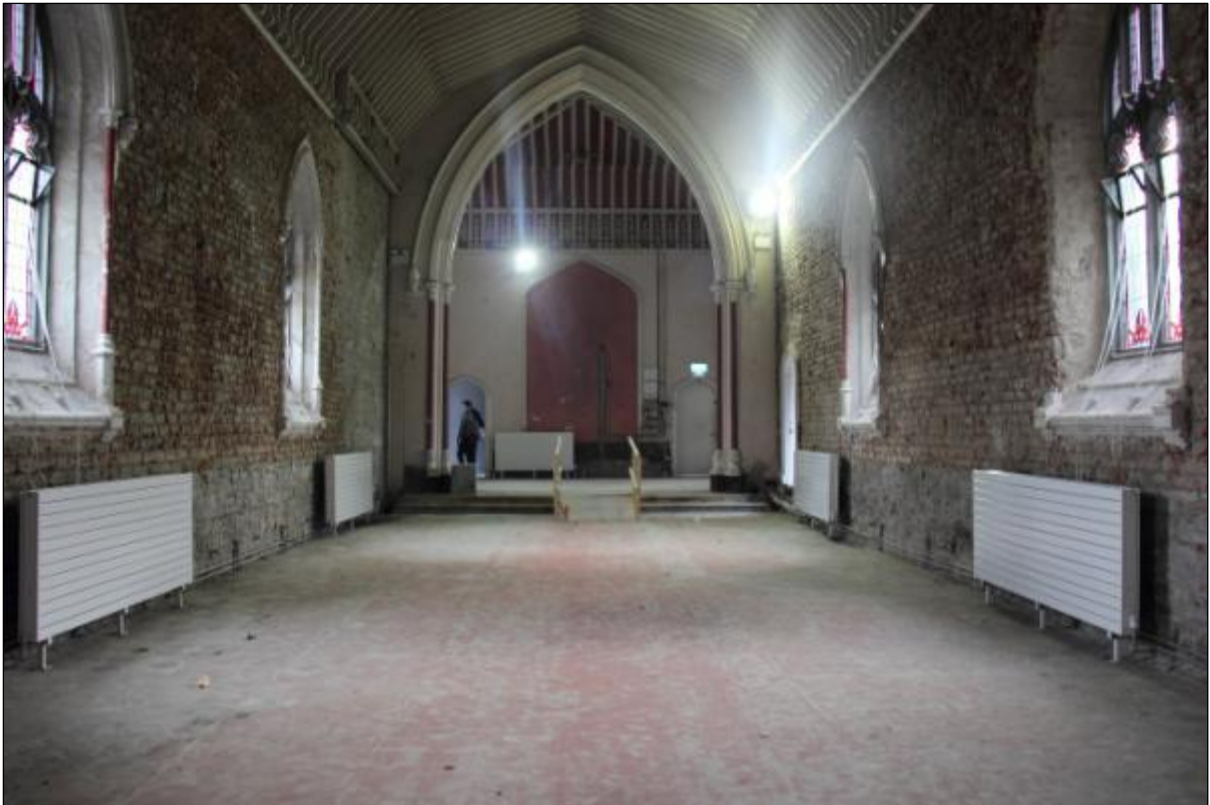
Photograph 112 Interior View of Chapel
