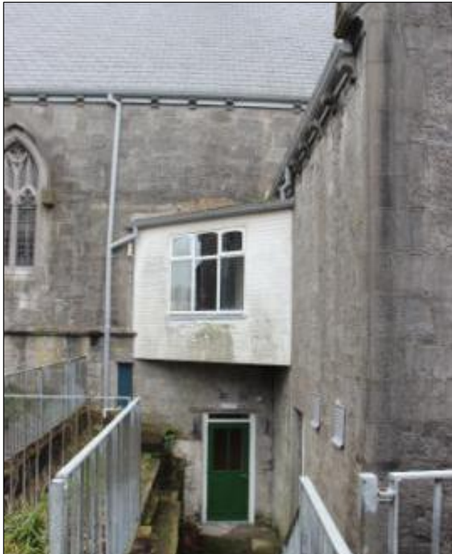
Photograph 109 Rear Elevation of Chapel showing timber extension
