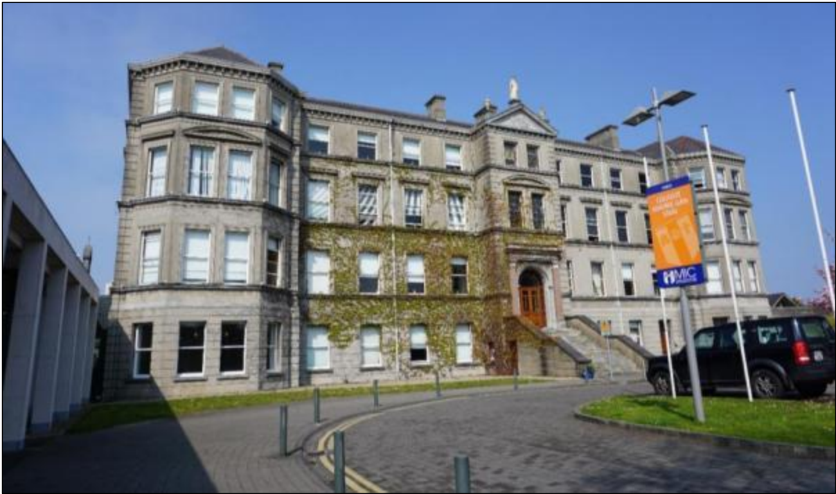
Photograph 64 Mary Immaculate College Foundation Building Front Elevation
