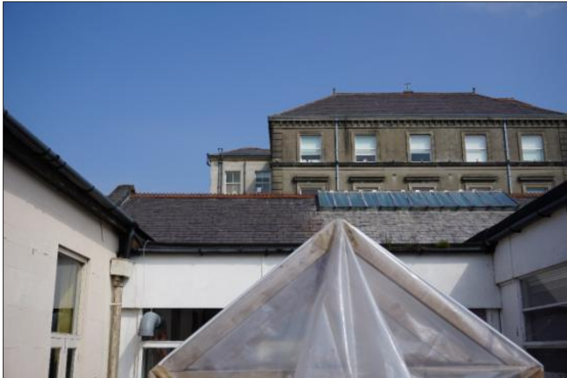
Photograph 77 External View of the recreational Hall showing natural slate roof.
