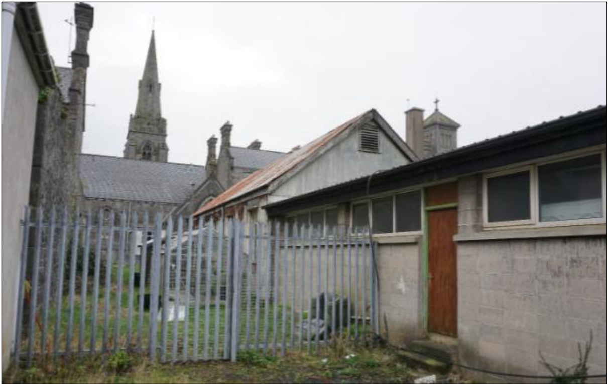
Photograph 115 Rear Elevation of Mount St. Vincent Hall
