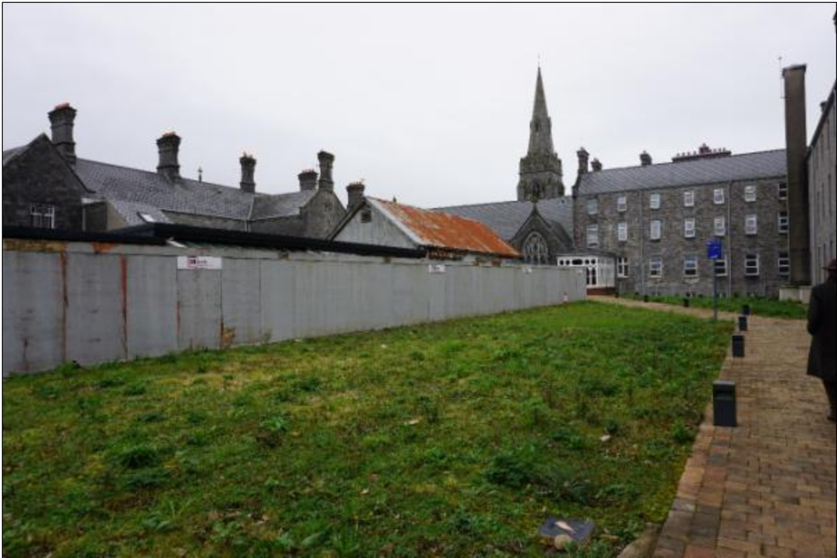
Photograph 113 Mount St. Vincent Hall surrounded by hoarding
