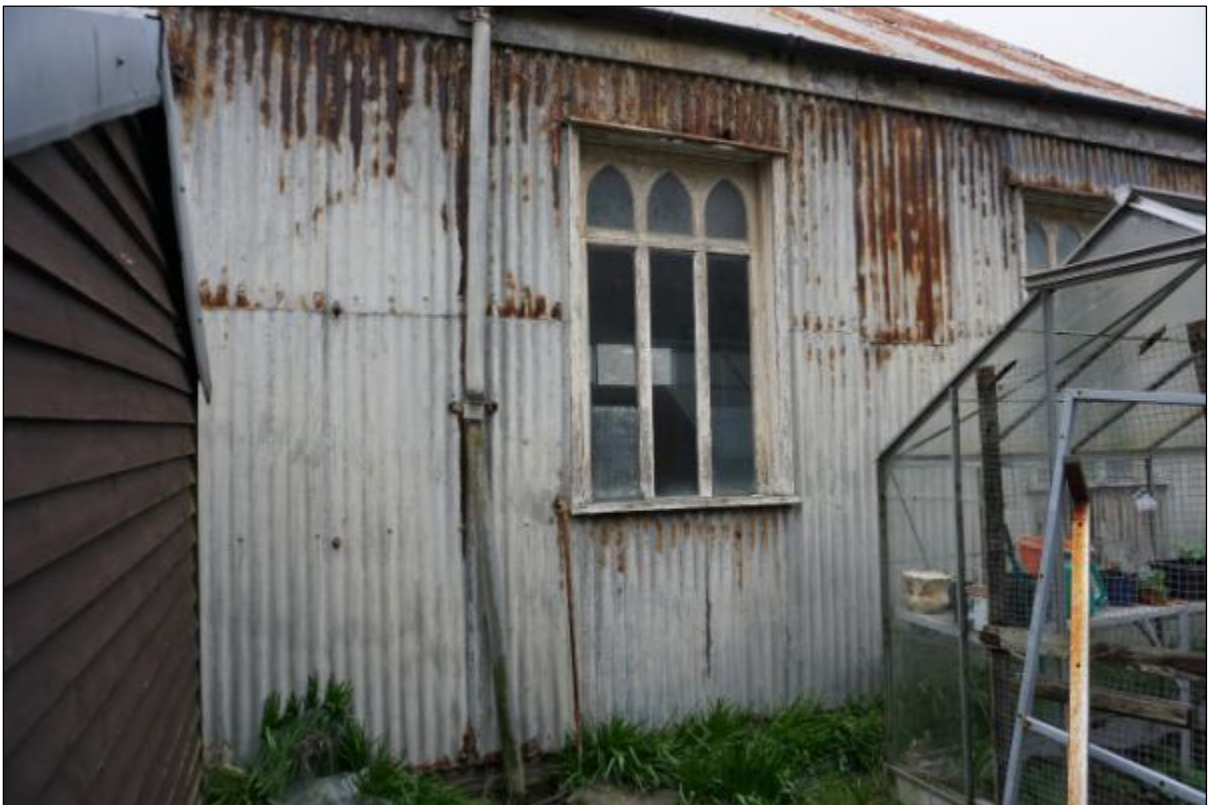
Photograph 116 Exterior View of window opening.
