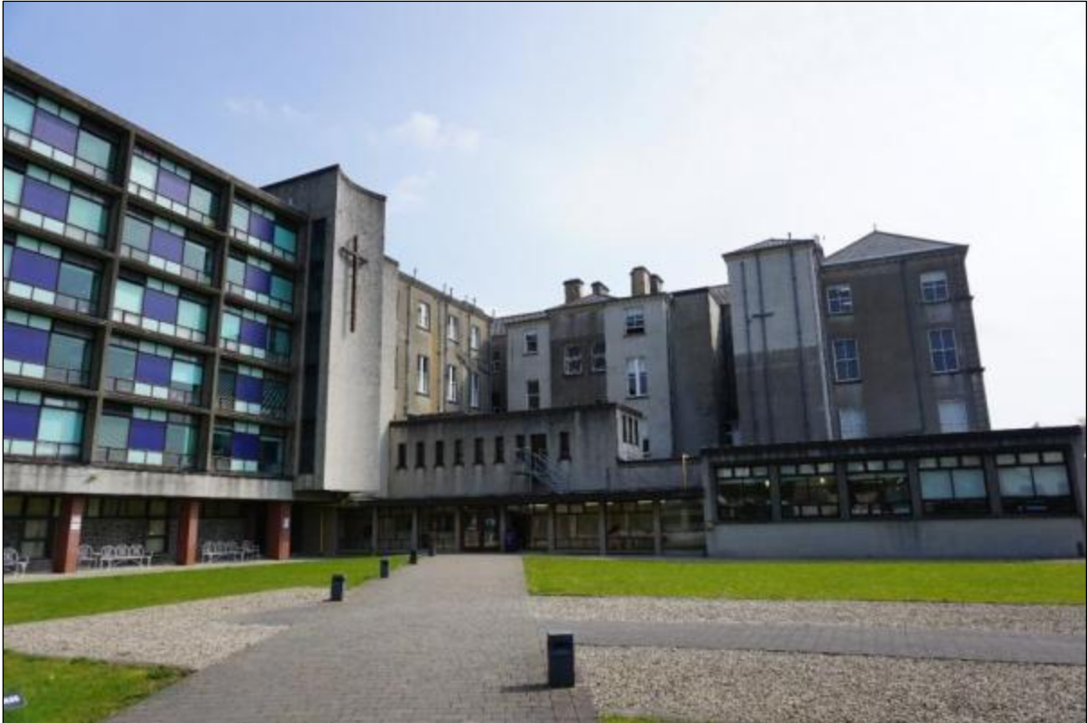
Photograph 66 Mary I Foundation Building Rear Elevation
