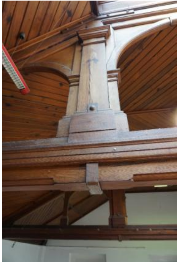
Photograph 79 Roof Structure Detail
