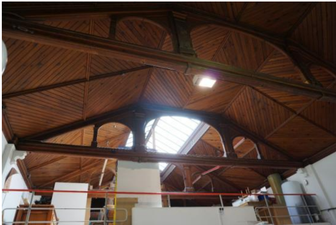
Photograph 78 Internal View of the recreational Hall showing Hammerbeam Roof and Mezzanine Level
