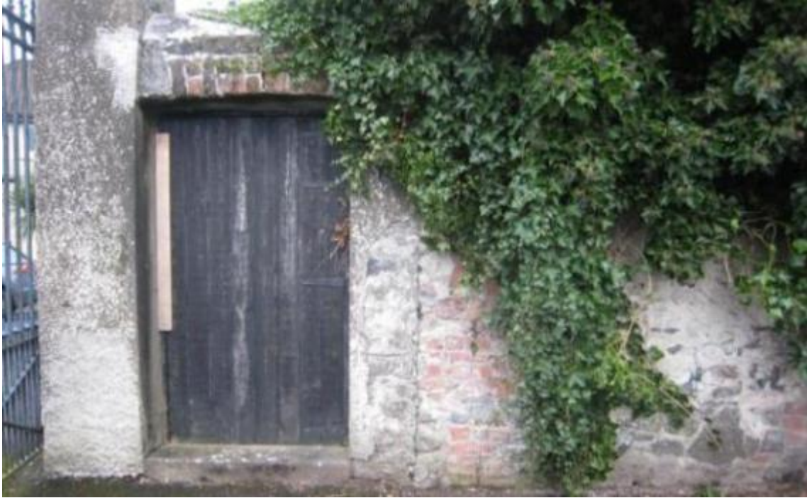
Photograph 58 Section of remaining 1840-1870 additions to the walled garden and entrance to Summerville House
