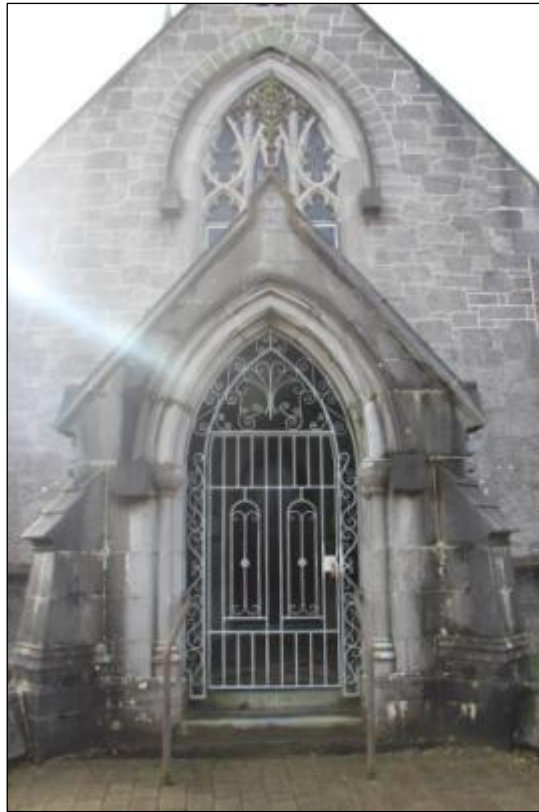
Photograph 110 Chapel Entrance porch
