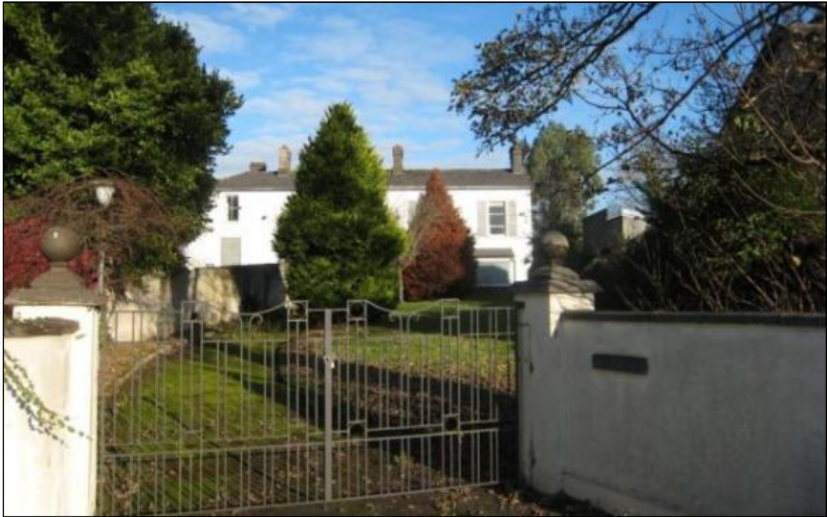
Photograph 37 Richmond House - entrance to the eastern property and the dividing wall is visible.
