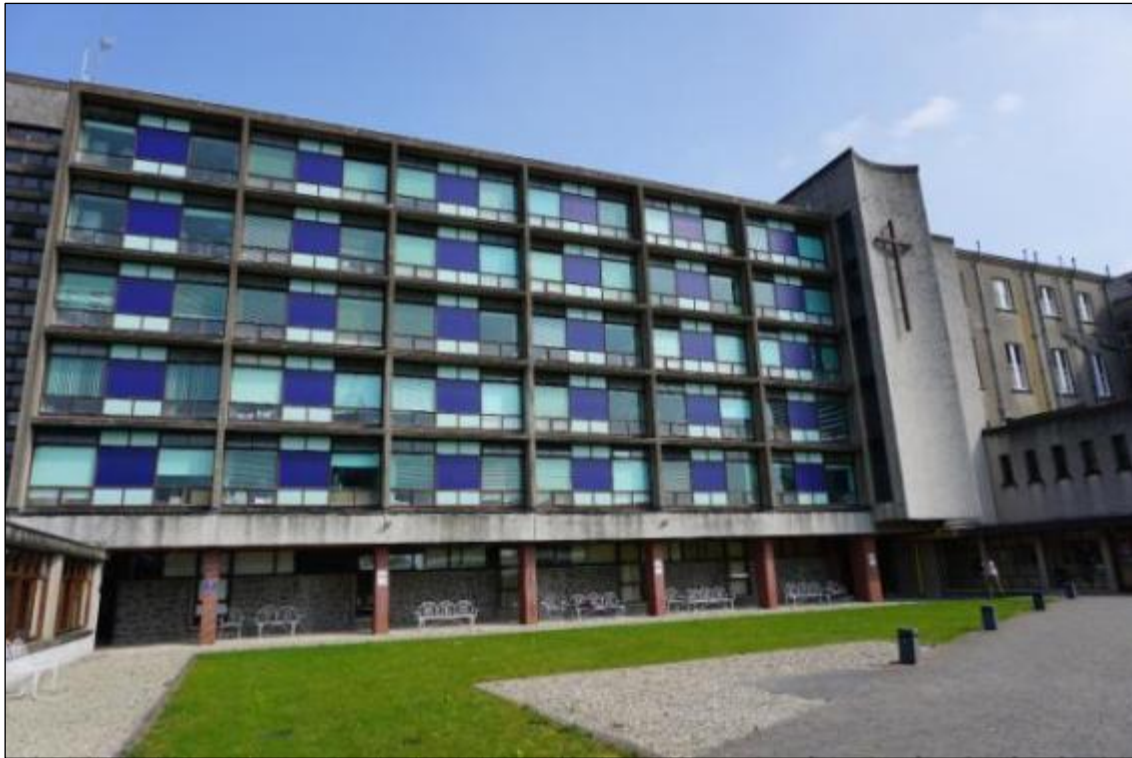
Photograph 83 Side elevation from Courtyard
