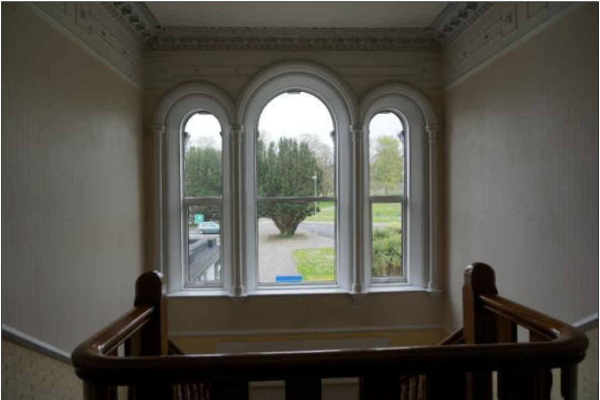
Photograph 93 Internal view of arch window openings at the top of the stairs
