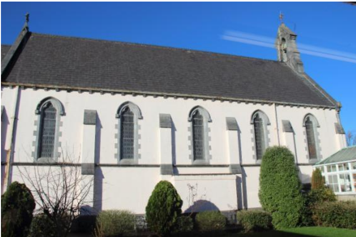
Photograph 71 Chapel, East Elevation showing Confessional
