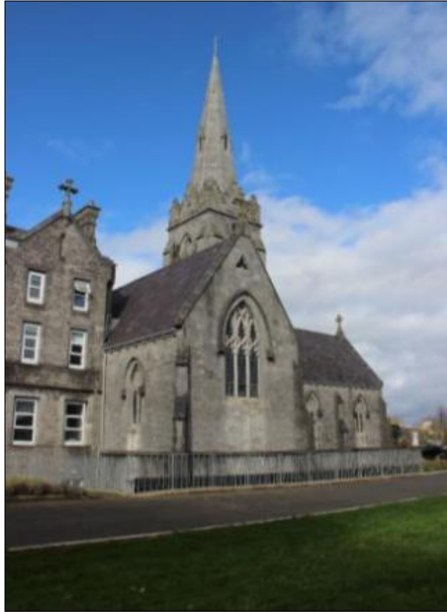
Photograph 108 Mount St Vincent Chapel Front Elevation
