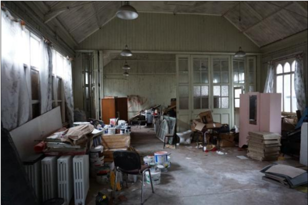
Photograph 117 Interior View showing folding doors
