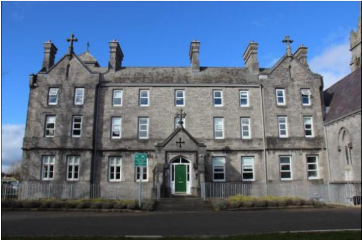
Photograph 101 Mount St. Vincent Front Elevation
