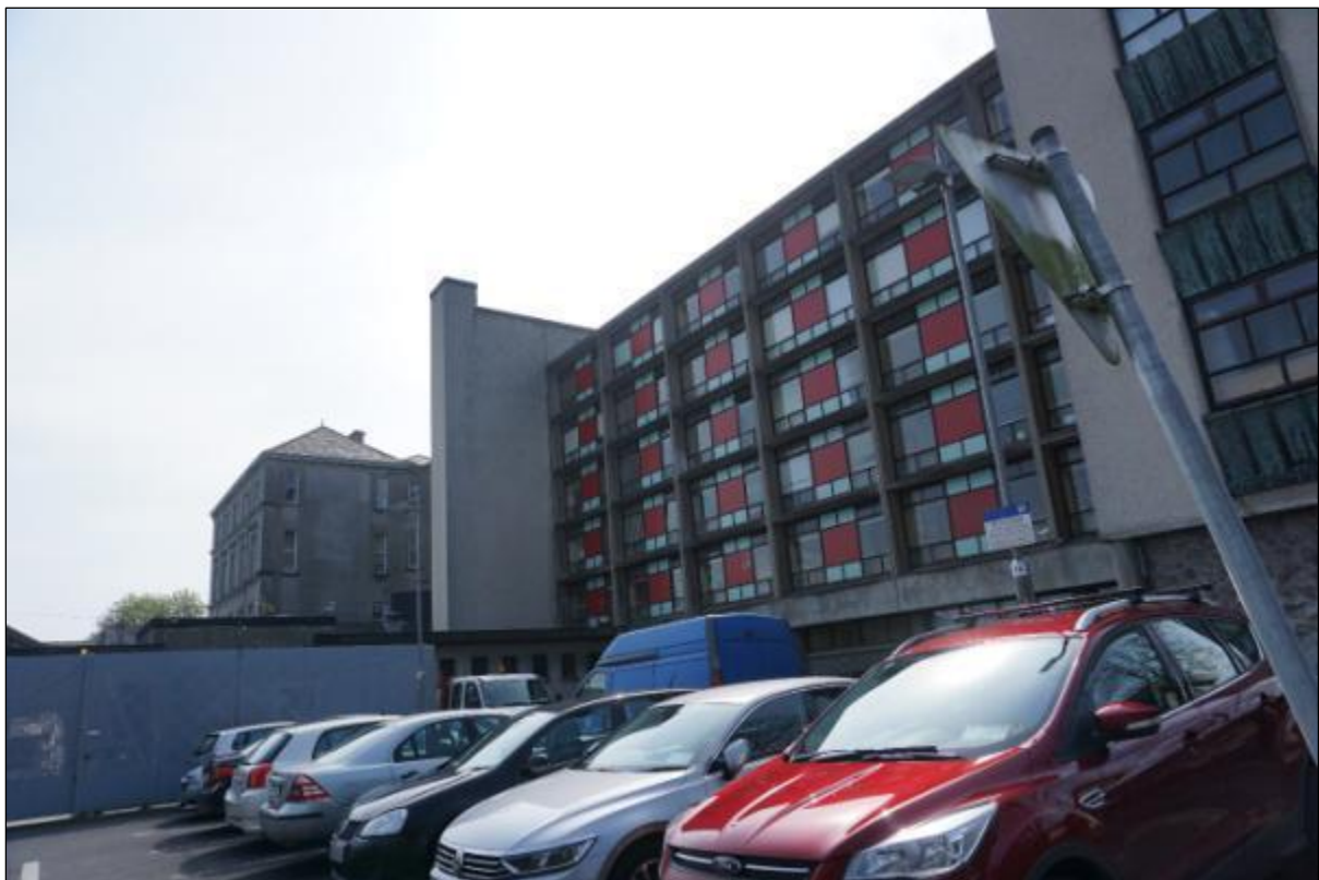
Photograph 80 Residential Block side elevation
