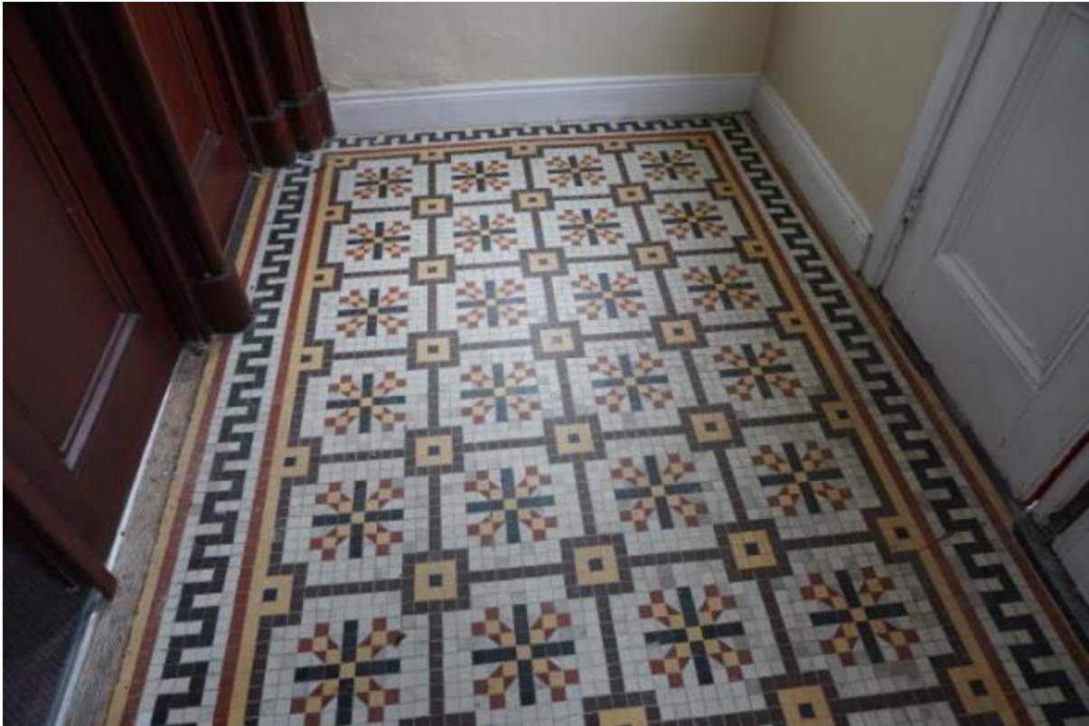
Photograph 95 Encaustic tile floor in Entrance Porch
