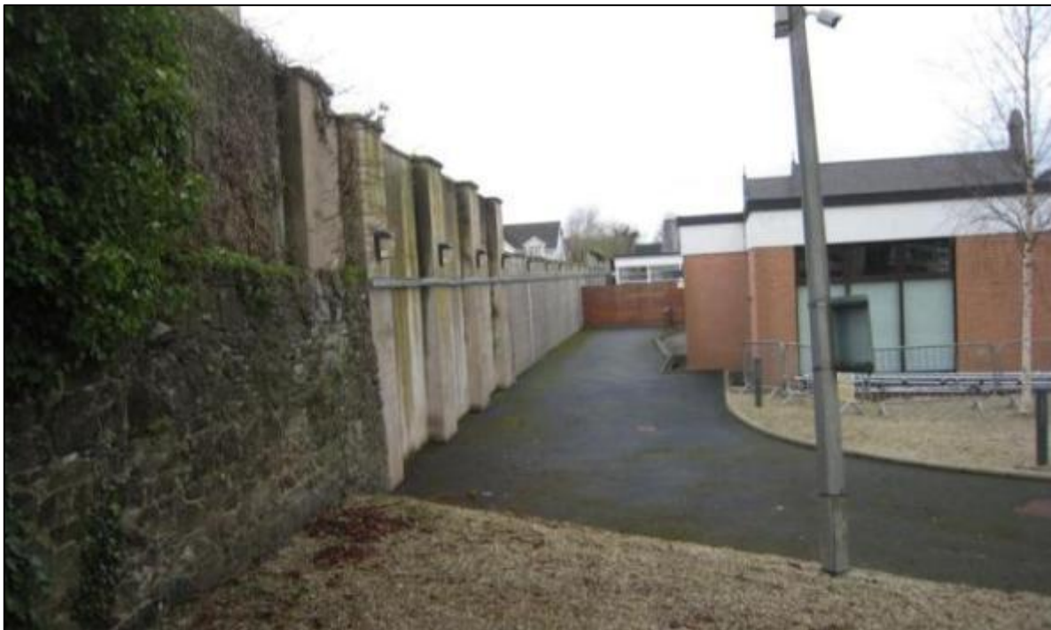
Photograph 45 Southern boundary line of Prospect House
