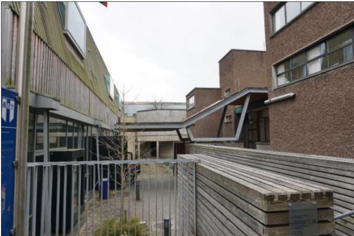
Photograph 15 Canopy connecting Library with TARA building
