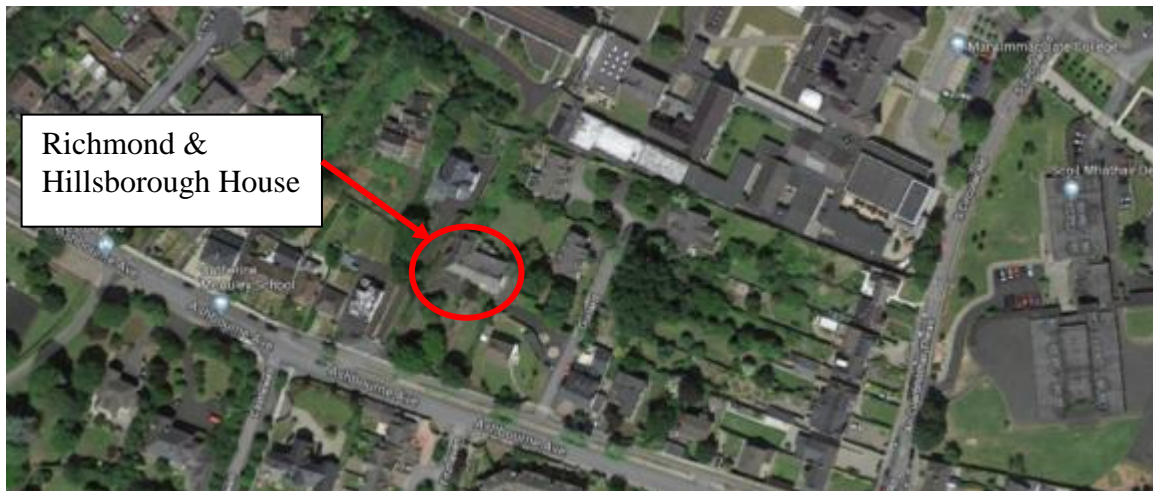
Figure 14 Aerial View of Richmond and Hillsborough House
